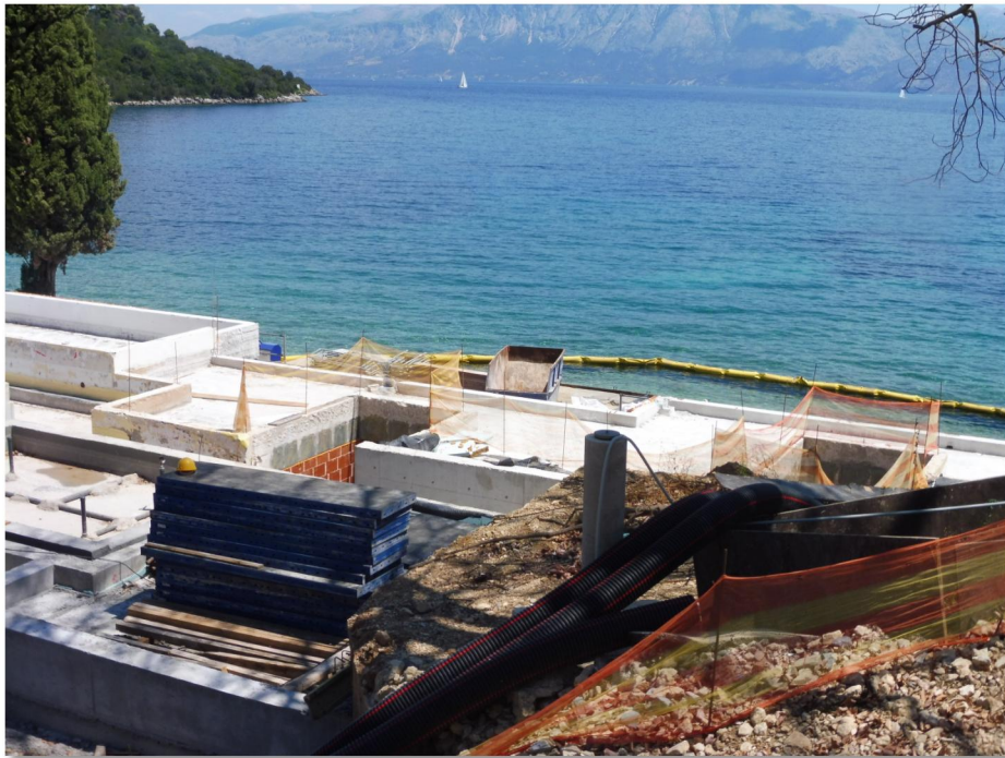
Figure 2.1-9. Marking of the project's working spaces with suitable fences.
