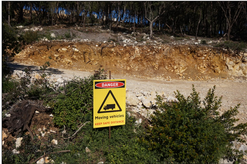
Figure 2.1-11. Warning signs for the movement of the vehicles throughout all the construction sites.
