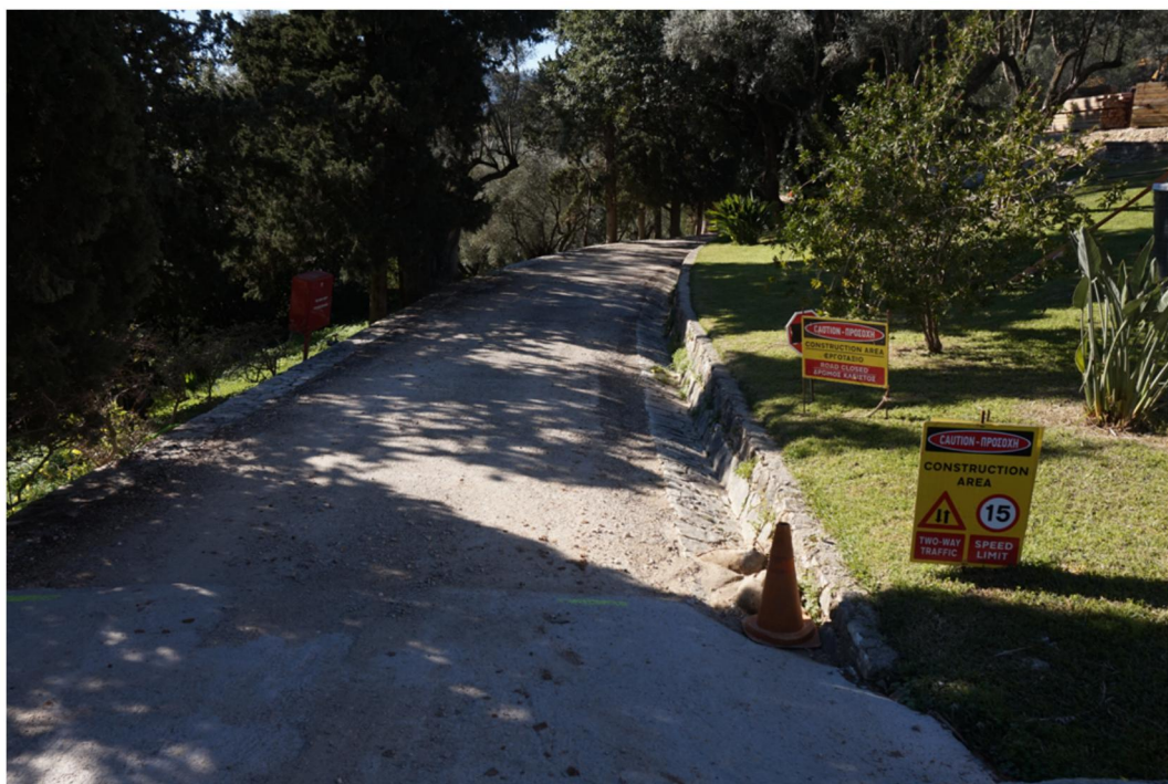
Figure 2.1-5: Speed limit up to 15km/h on non-paved roads or roads in bad condition.
