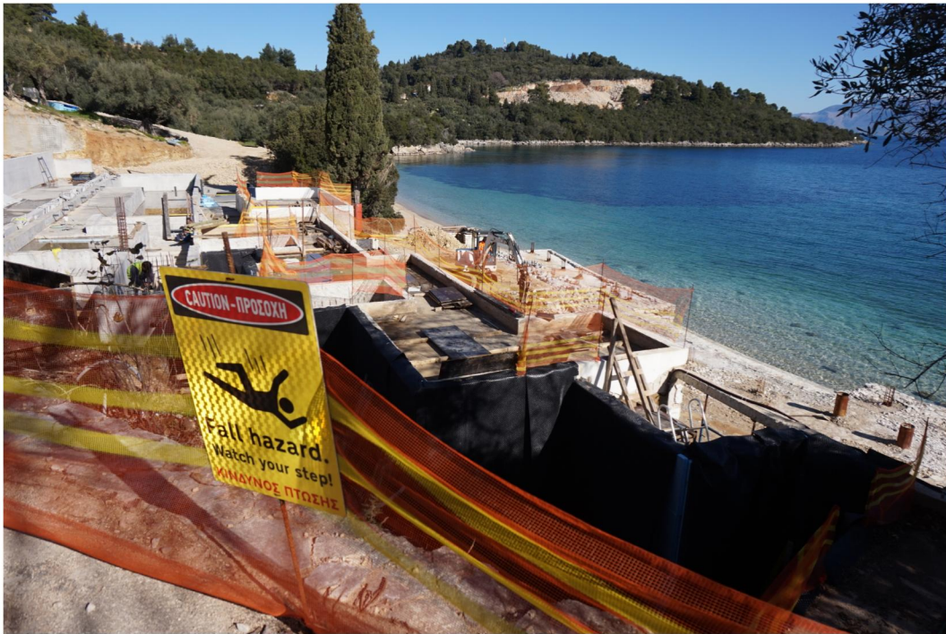
Figure 2.1-4: Warning signs and protective net at every construction site.
