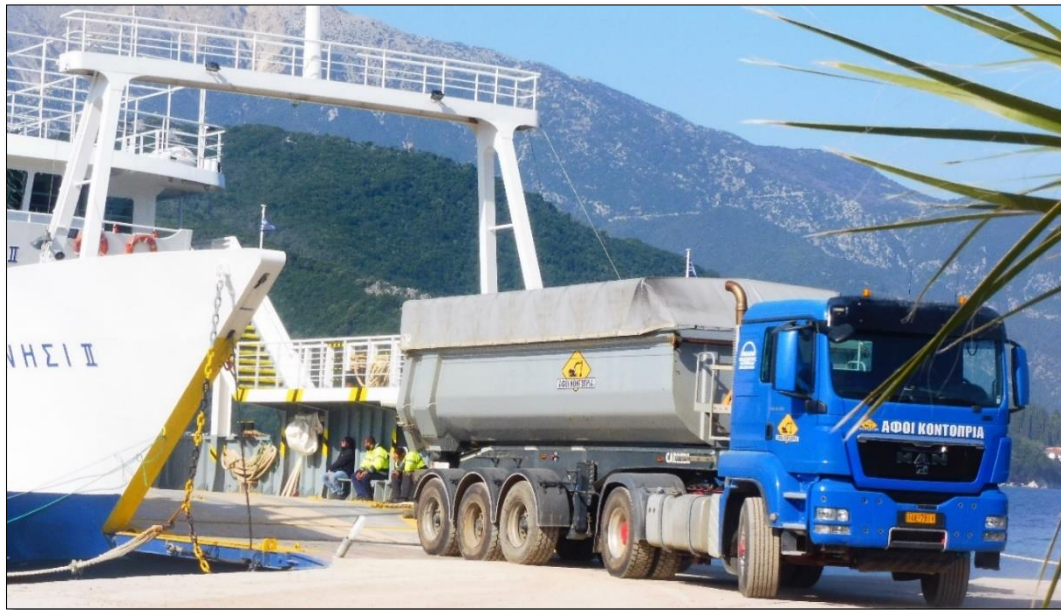
Figure 2.1-5: Excavation material transport with Covered trucks.
