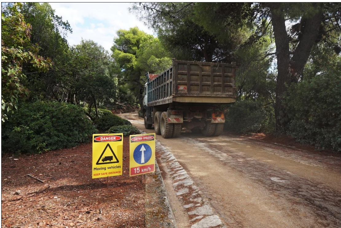
Figure 2.1-3: Truck commuting from excavation area to construction sites.
