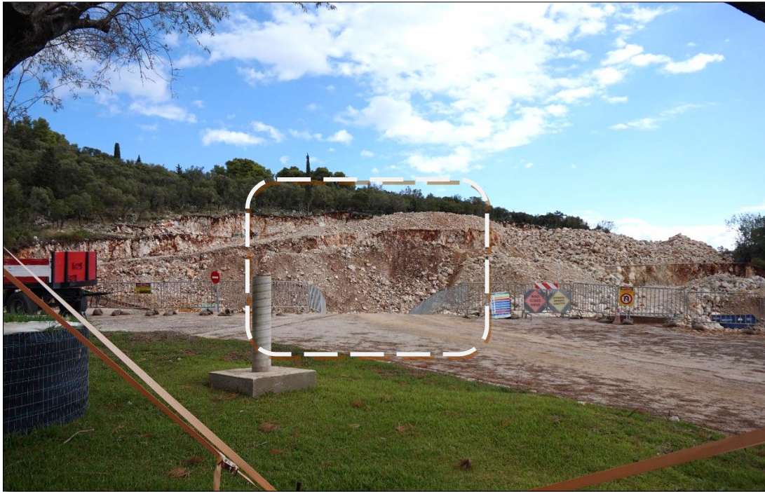
Figure 2.2-3: Local construction site during micro-blast procedure. No dust emissions present.
