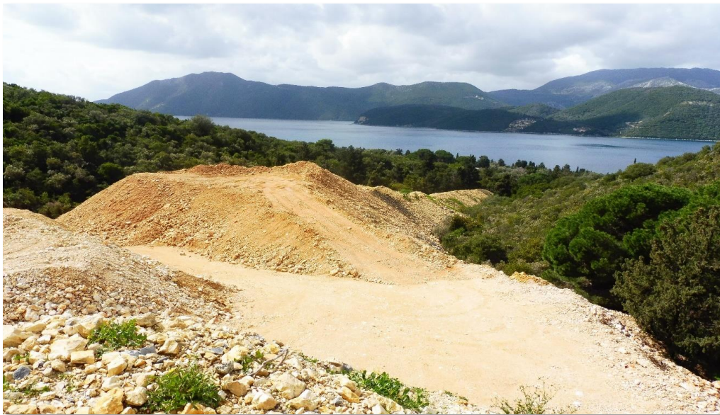
Figure 2.1.3-2. View from the Incinerator construction site.
