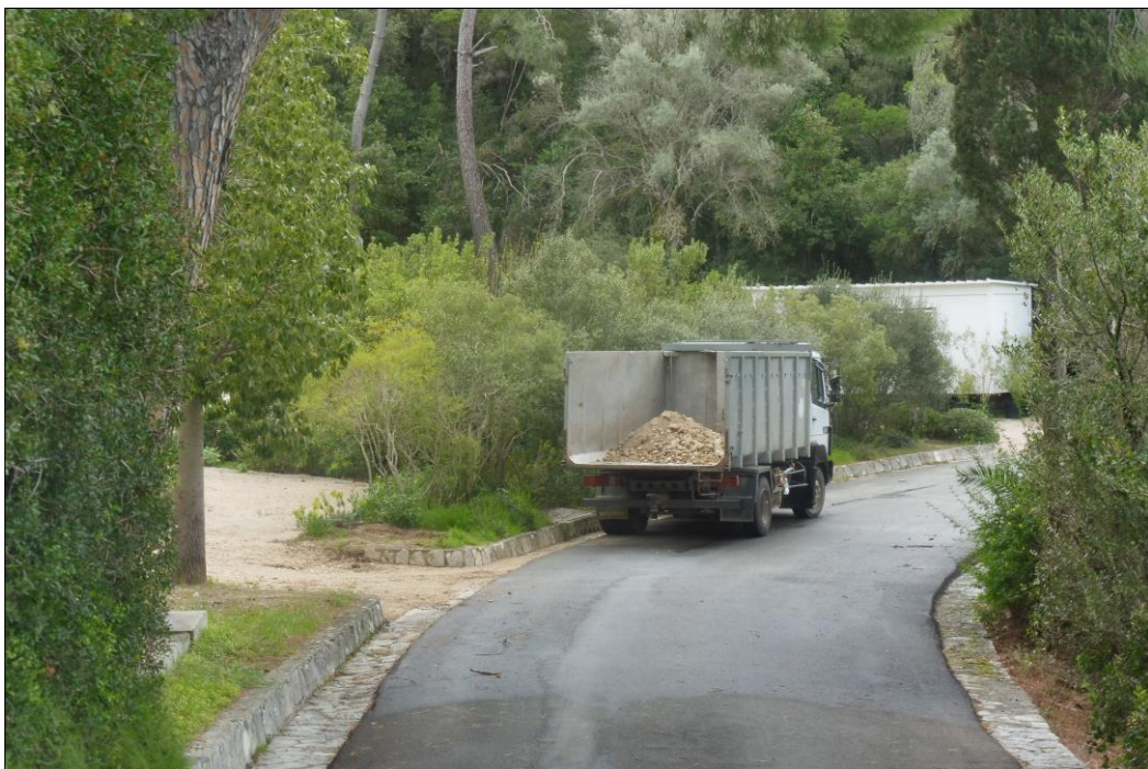
Figure 2.1.2-1. Truck load noticed without the appropriate lining.
