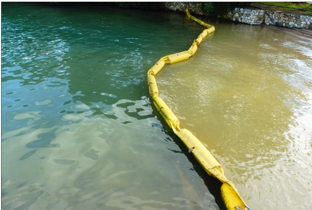
Figure 2.3-1: Silt curtain in place for protection near a coastal construction site.
